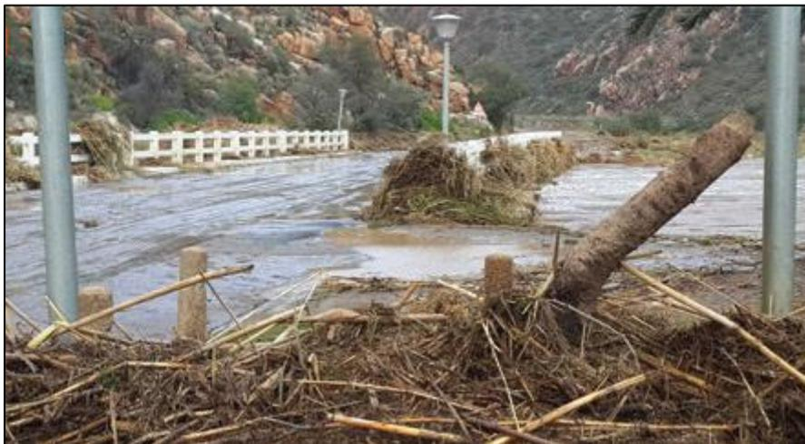
**Figure 20: Debris clogging Voortrekker Bridge leading into Montagu during the 2015 flood (Source: Patrick O'Shea in Pharoah et al. 2016)**
