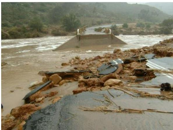
**Figure 11a: Bridge and road damage in die Kogmanskloof during the 2003 COL (Source: CWDM 2018)**
