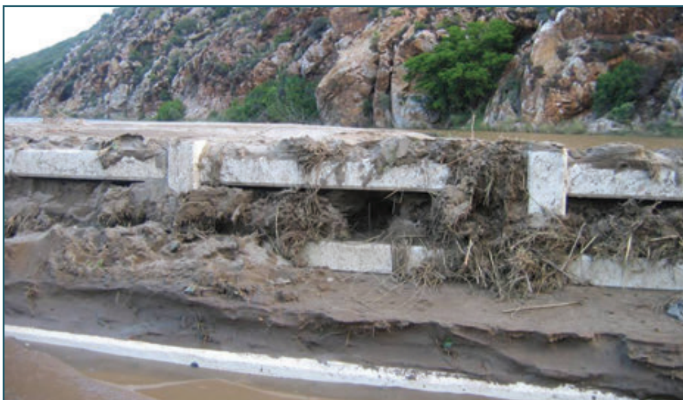
Figure 2.3.2.4: Debris blocking Voortrekker Bridge in Montagu (Source: Jan Durand)
