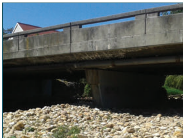
Figure 2.3.2.2: Aggradation beneath the Andreas Pretorius Bridge, Somerset West (Source: IWEE, 2014)
