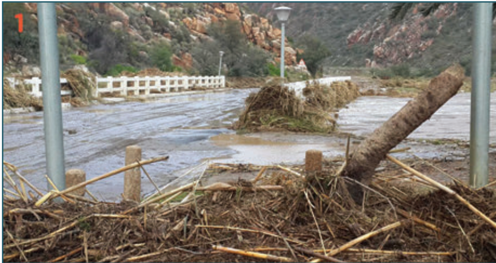
Figure 2.3.2.3: Debris clogging a bridge leading into Montagu (Source: Patrick O’Shea, Adverteyes: http://montagudriedfruitnuts.co.za/montagu-floods-june-2015-keisie-kingna-rivers/ )
