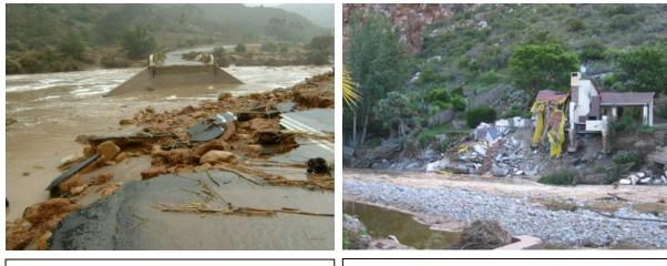
Figure 11a: Bridge and road damage in die Kogmanskloof during the 2003 COL (Source: CWDM 2018)
