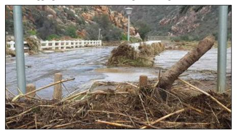
Figure 20: Debris clogging Voortrekker Bridge leading into Montagu during the 2015 flood (Source: Patrick O'Shea in Pharoah et al. 2016)
