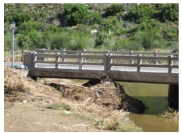
Figure 9: Aggradation beneath the Voortrekker Bridge, Montagu (Source: Jan Durand in Pharoah et al. 2016)
