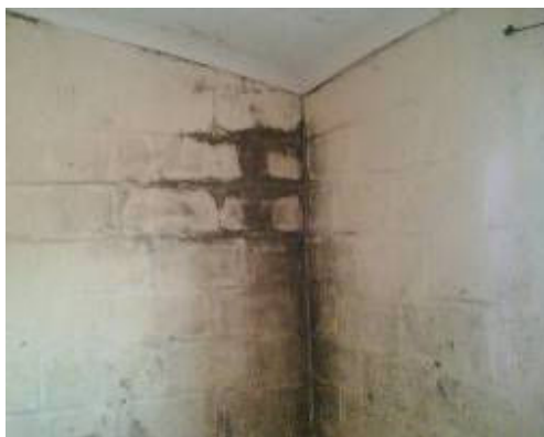
Figure 3.2.3.2.14: Damp and mouldy wall inside RDP dwelling
