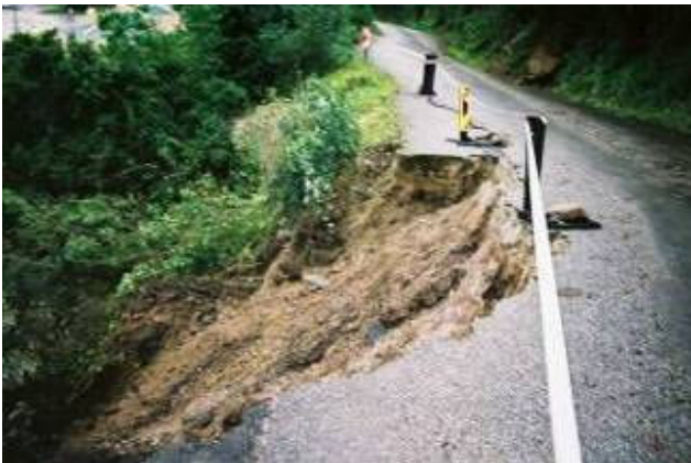
Figure 2.3.4.2.6: Significant damage to a road due to slope failure (mass movement) underneath the road
