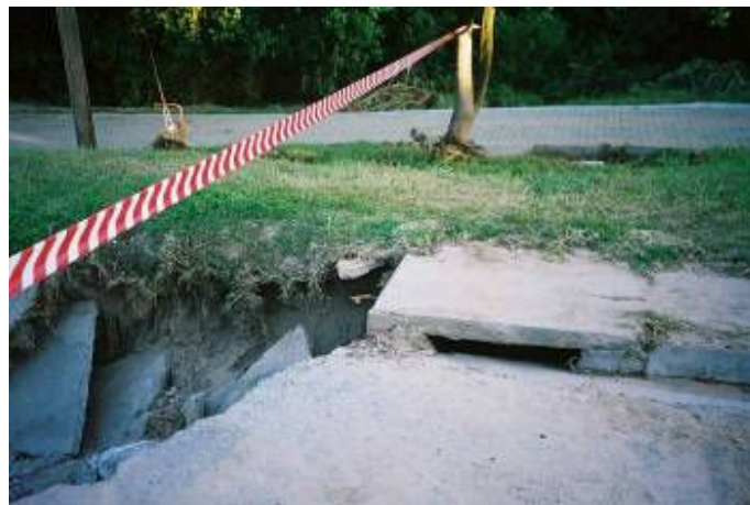
Figure 2.3.4.3.6: The storm water drainage system was unable to cope with the surface run-off
