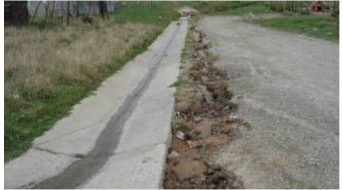
Figure 3.2.3.1.5: Sloping tarred road eroded by run-off
