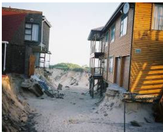
Figure 3.2.7.2.7: Houses destabilised and partially collapsed because of storm water run-off
