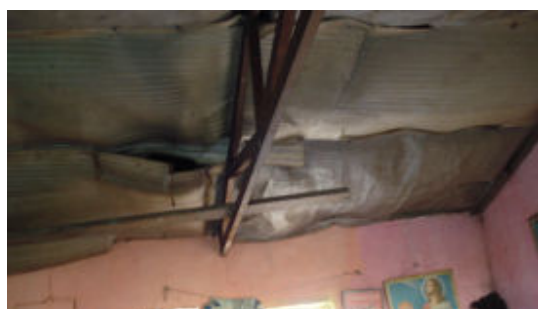
Figure 3.2.3.2.10: Debilitated roof of RDP dwelling sagging from rainwater
