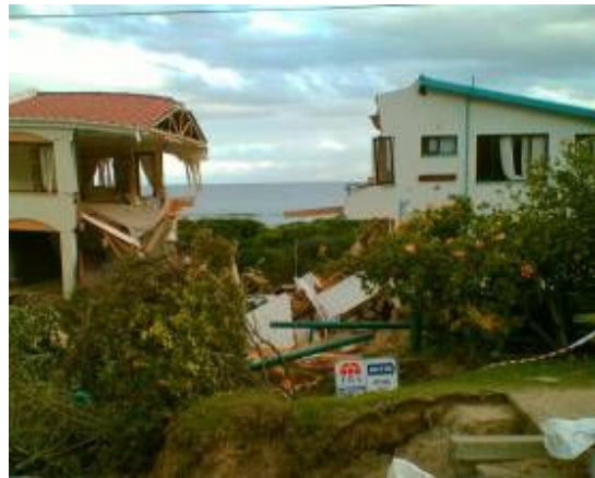
Figure 3.2.7.2.6: House collapsed because of storm water run-off destabilising its foundation
