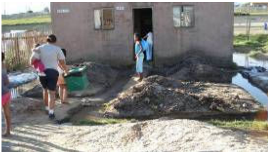
Figure 3.2.3.2.8: Run-off from street entering RDP through front door
