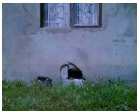
Figure 3.2.3.2.3: A hole made in an RDP dwelling to drain out water
