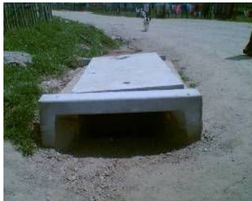
Figure 3.4.3: Newly installed storm water drain
