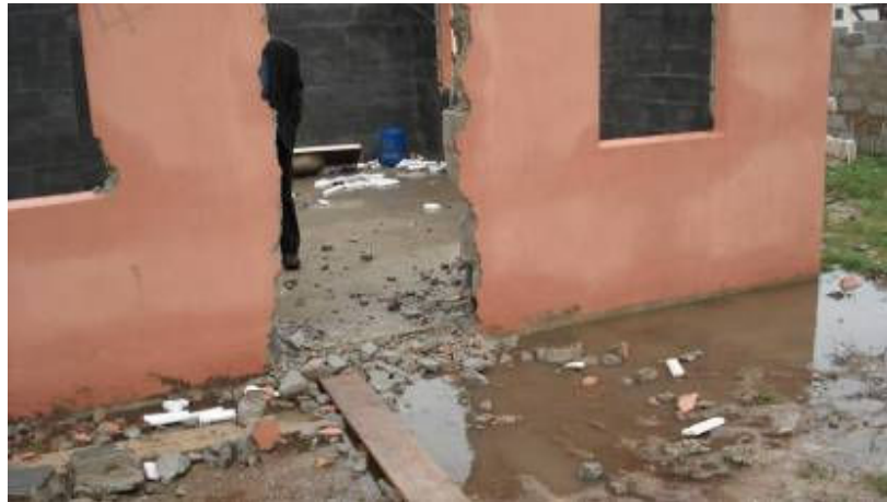
Figure 3.2.3.2.11: Part of the wall of a RDP house washed away by storm water run-off
