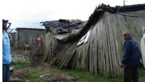
Figure 3.2.3.2.1: A seriously affected informal dwelling, located in a poorly drained area with high water table
