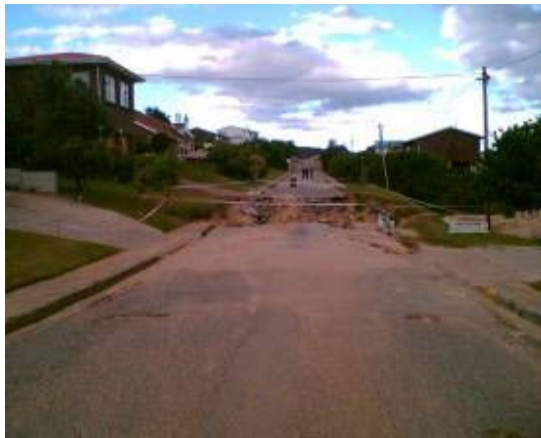
Figure 3.2.7.2.5: Road collapsed because storm water drain burst
