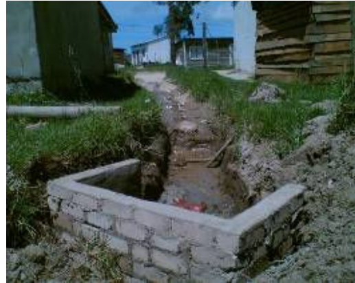
Figure 3.4.2: Newly installed storm water culvert and channel, although incomplete
