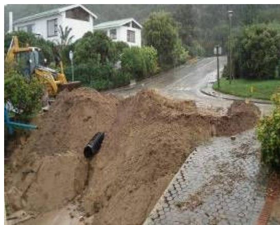
Figure 3.2.7.2.8: Road damaged because of storm water overflowing
