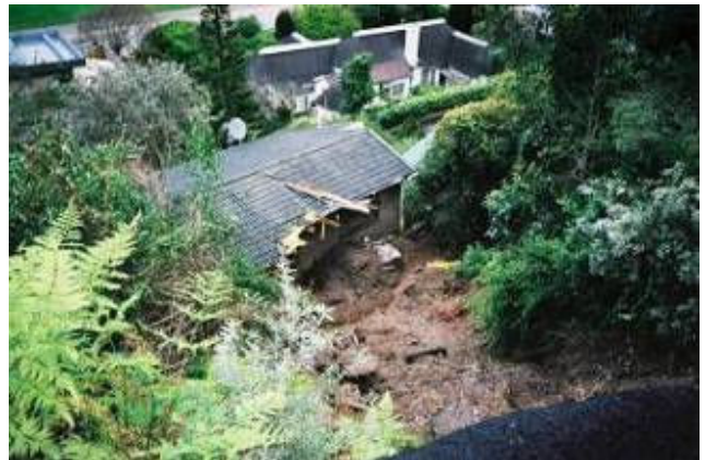
Figure 2.3.4.2.7: Significant damage to a house, due to slope failure (mass movement) underneath the road
