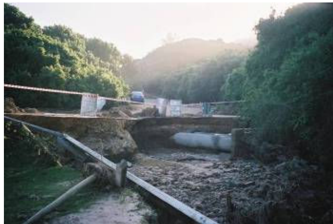
Figure 2.3.4.3.9: A 4 metre wide gully formed along the side of a road
