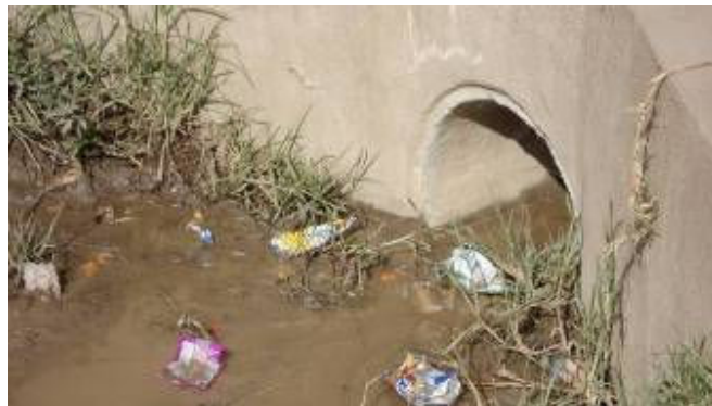
Figure 3.2.3.1.6: Storm water outlet onto road
