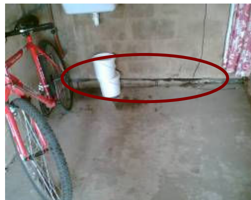
Figure 3.2.3.2.15: Subsided foundation because of high water table
