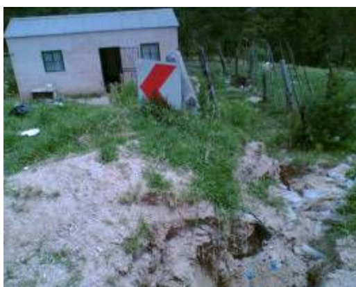
Figure 3.2.3.1.7: Storm water outlet running directly towards RDP house
